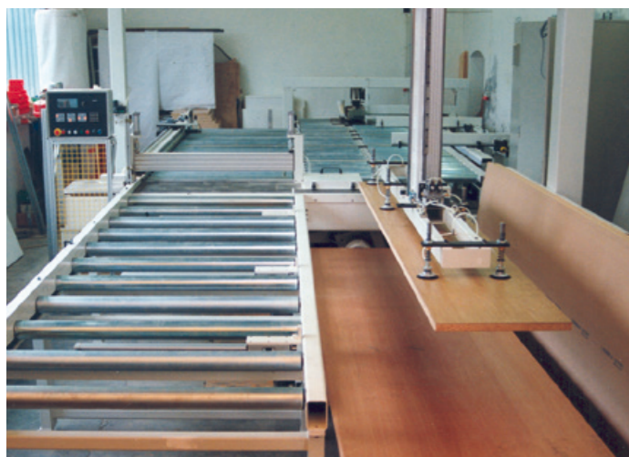
Board pre-cut saw
